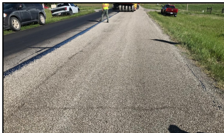
Top: Spreader placing chip seal aggregate Bottom: Completed chip sealing
