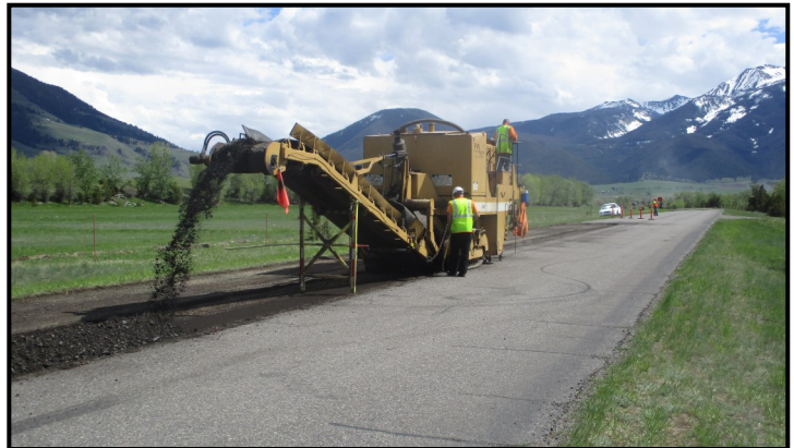
Top: Roadway reconditioning in gravel road section
