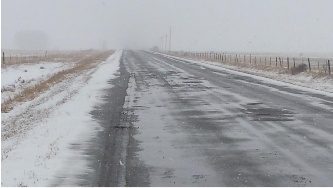
5. Typical area of pothole repair in centerline, travel lanes and shoulder.
