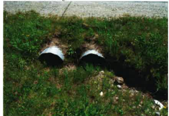
Silver Gate - culverts at south end of park
