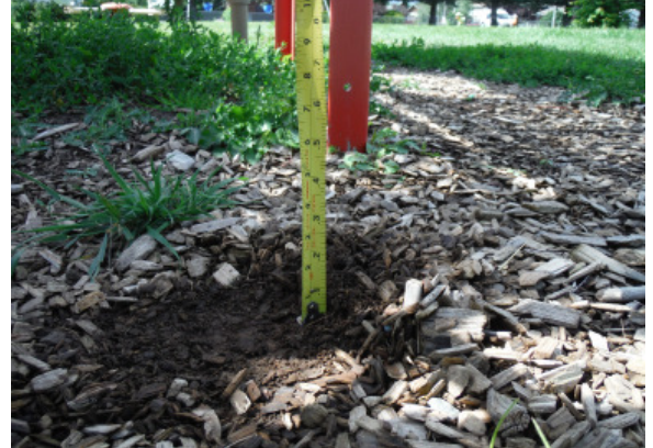
Green Acres - essentially non-existent fall surfacing
