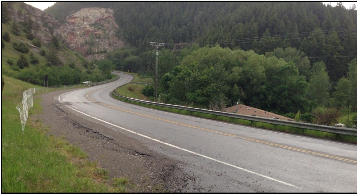
Photo 43. Looking south at insufficient sight distance due to vertical and horizontal curves on MT 86 at the access to “M” trail parking lot. RP 4.2.
