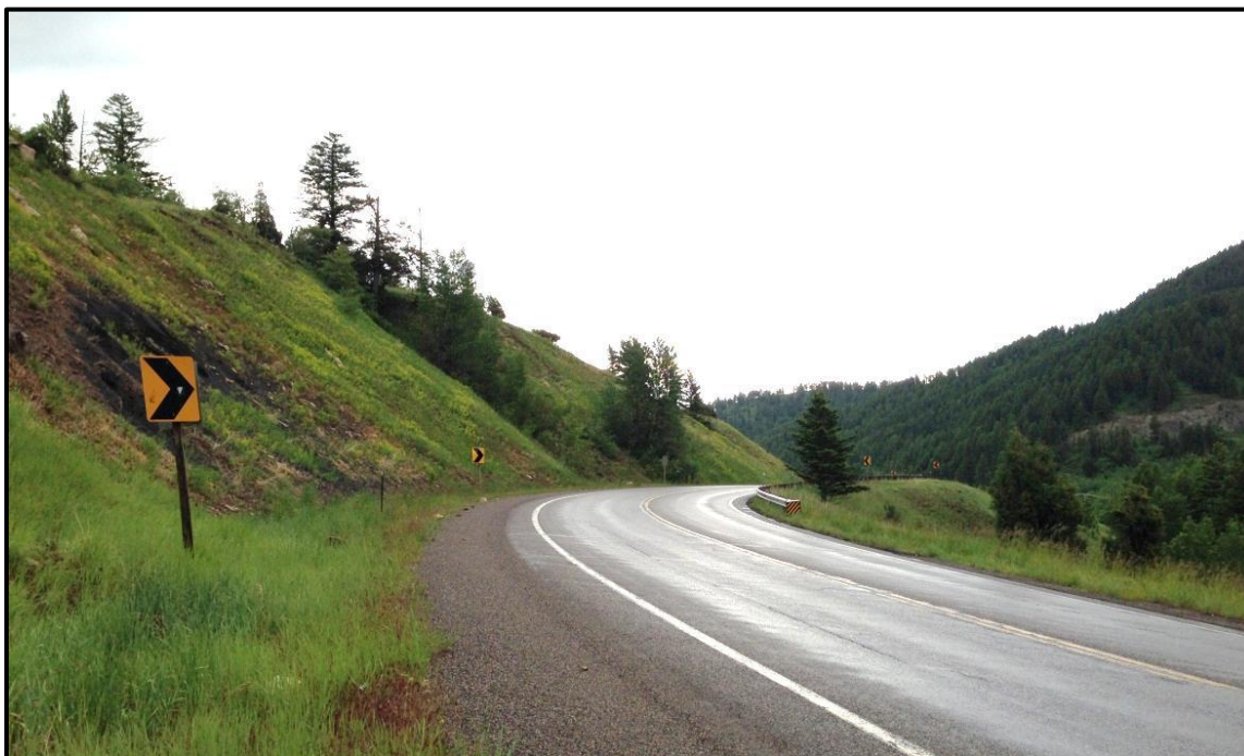
Photo 49. Looking at insufficient sight distance due to horizontal curves on MT 86. Substandard back slopes are also visible. RP 4.6.
