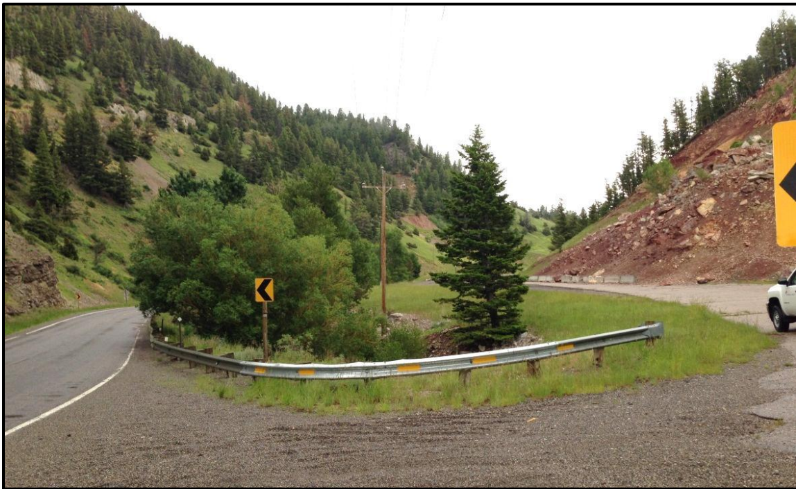
Photo 46. Looking north at insufficient sight distance due to horizontal curves and natural features on MT 86 at the access to the old highway looking east. RP 4.4.
