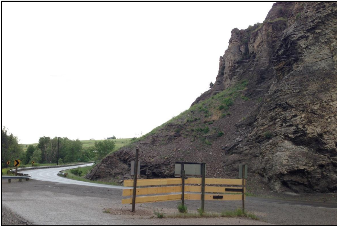
Photo 45. Looking at insufficient sight distance due to horizontal curves and natural features on MT 86 at the access to the old highway. RP 4.4.
