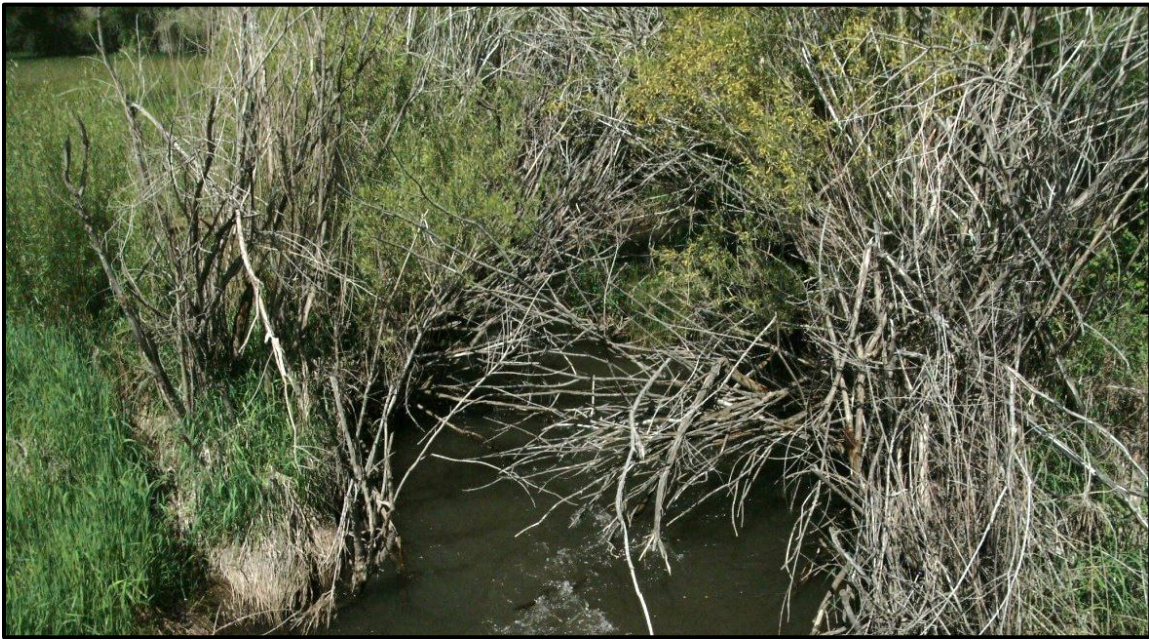
Photo 29. Looking upstream (west) on MT 86 crossing of Carrol Creek. RP 28.0.
