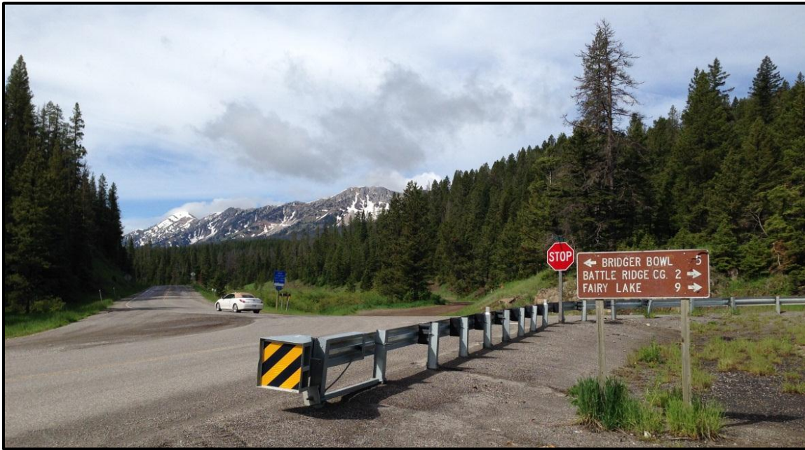
Photo 67. Looking at insufficient sight distance due to horizontal and vertical curves on MT 86 near Brackett Creek. RP 18.8.
