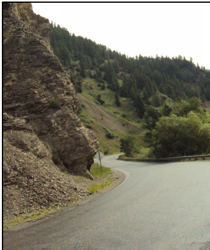
Photo 44. Looking north on MT 86, a rock outcropping is directly adjacent to the traveled way on the west side of the road. RP 4.4.
