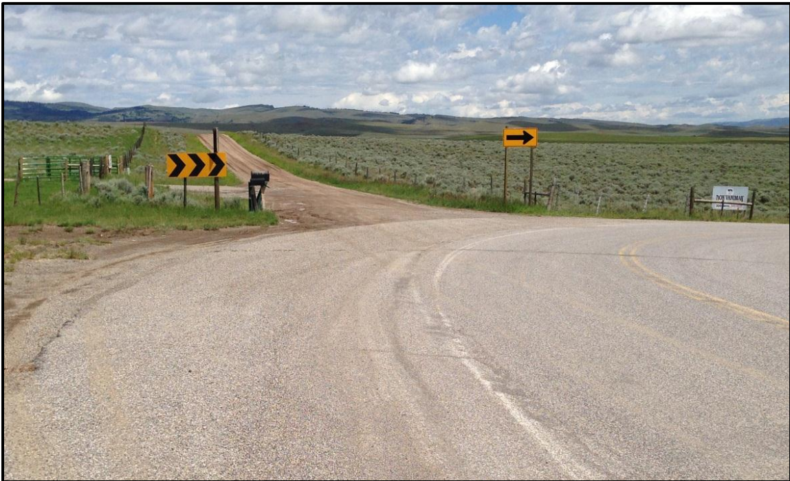
Photo 94. Looking at a tight horizontal curve on MT 86. RP 28.9.
