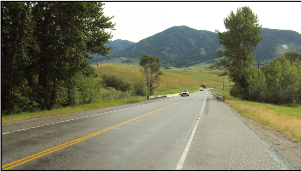
Photo 37. Looking north on MT 86 near the city limits of Bozeman. RP 3.0.
