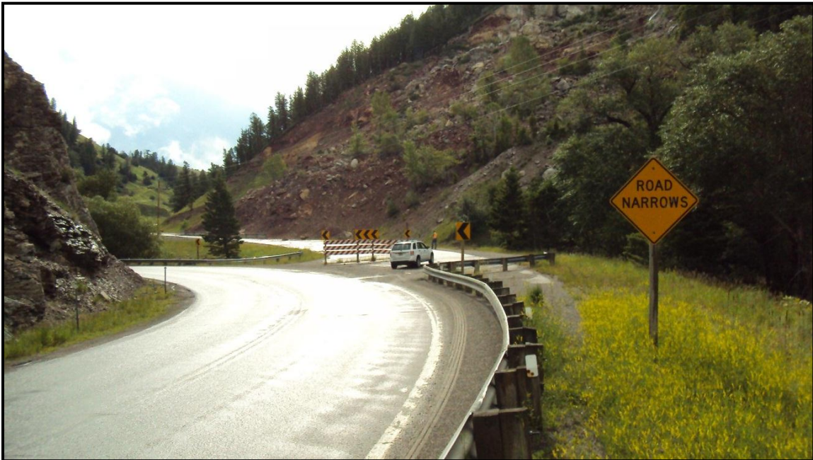
Photo 48. Looking north on MT 86, the roadway narrows with rock outcroppings along the west side of the road. RP 4.4.
