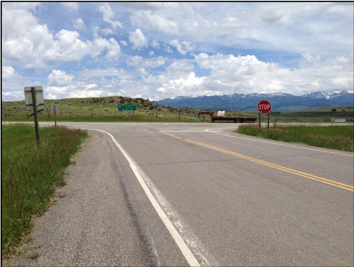
Photo 95. Looking east at the eastern/northern terminus of the corridor at the intersection of MT 86 and US 89. RP 37.5.
