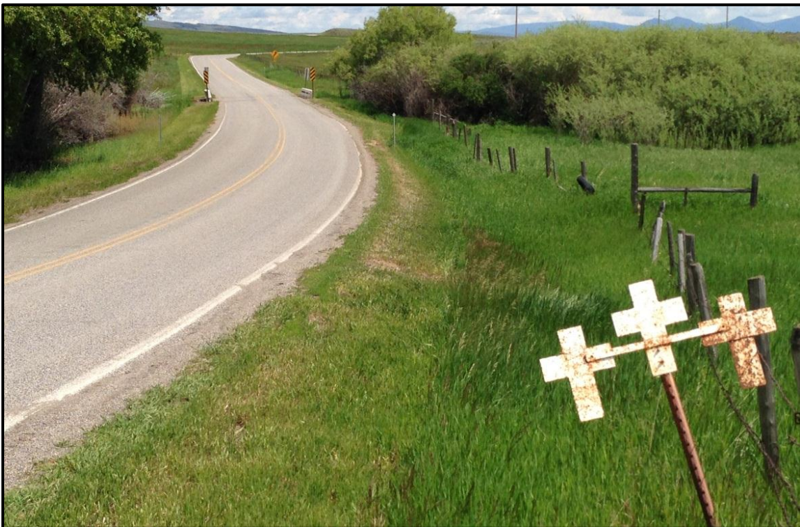
Photo 90. Looking north at insufficient sight distance due to horizontal and vertical curves on MT 86. RP 28.7.
