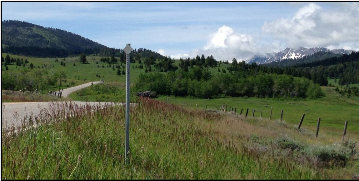
Photo 75. Looking at insufficient sight distance due to horizontal and vertical curves on MT 86. RP 24.5.
