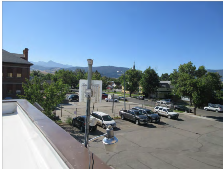
FIGURE 5 9-1-1 Center to Meyers Flats Microwave Radio and Panel Antenna
