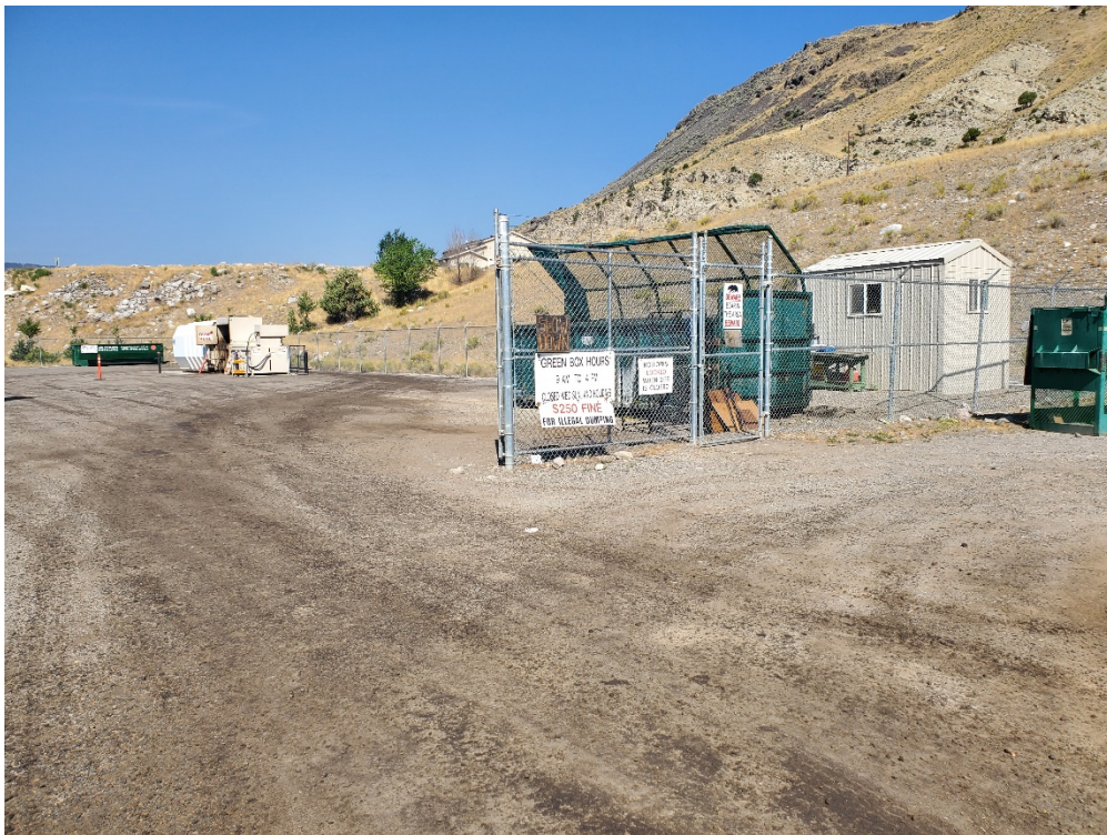
Gardiner Access Gate and Attendant Shack
