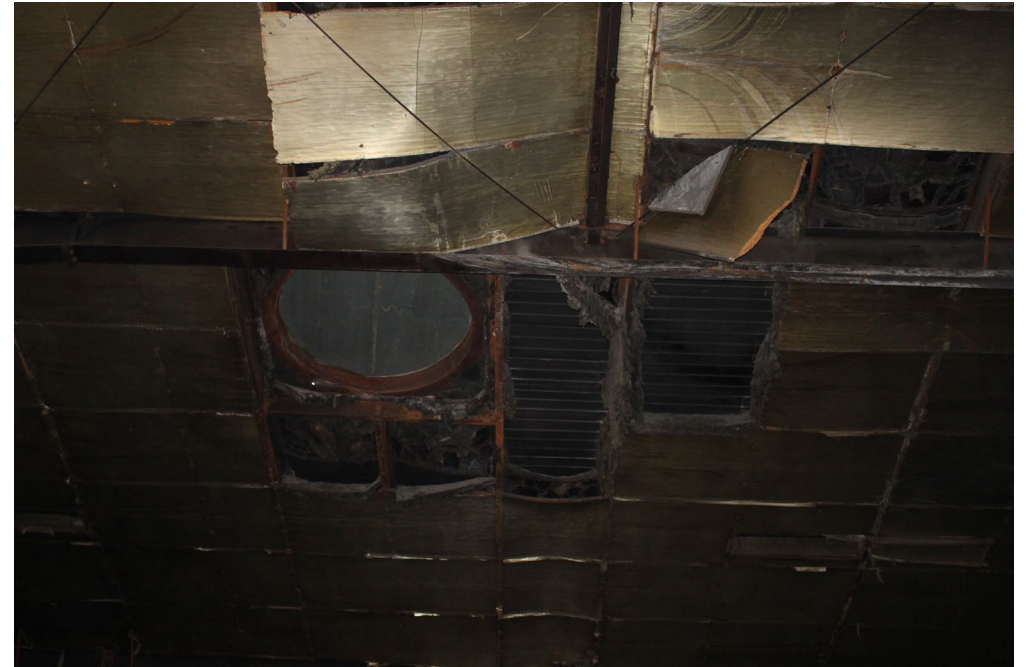
▲ Transfer Station Roof
