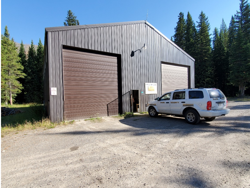
Cooke City Solid Waste Transfer Building
