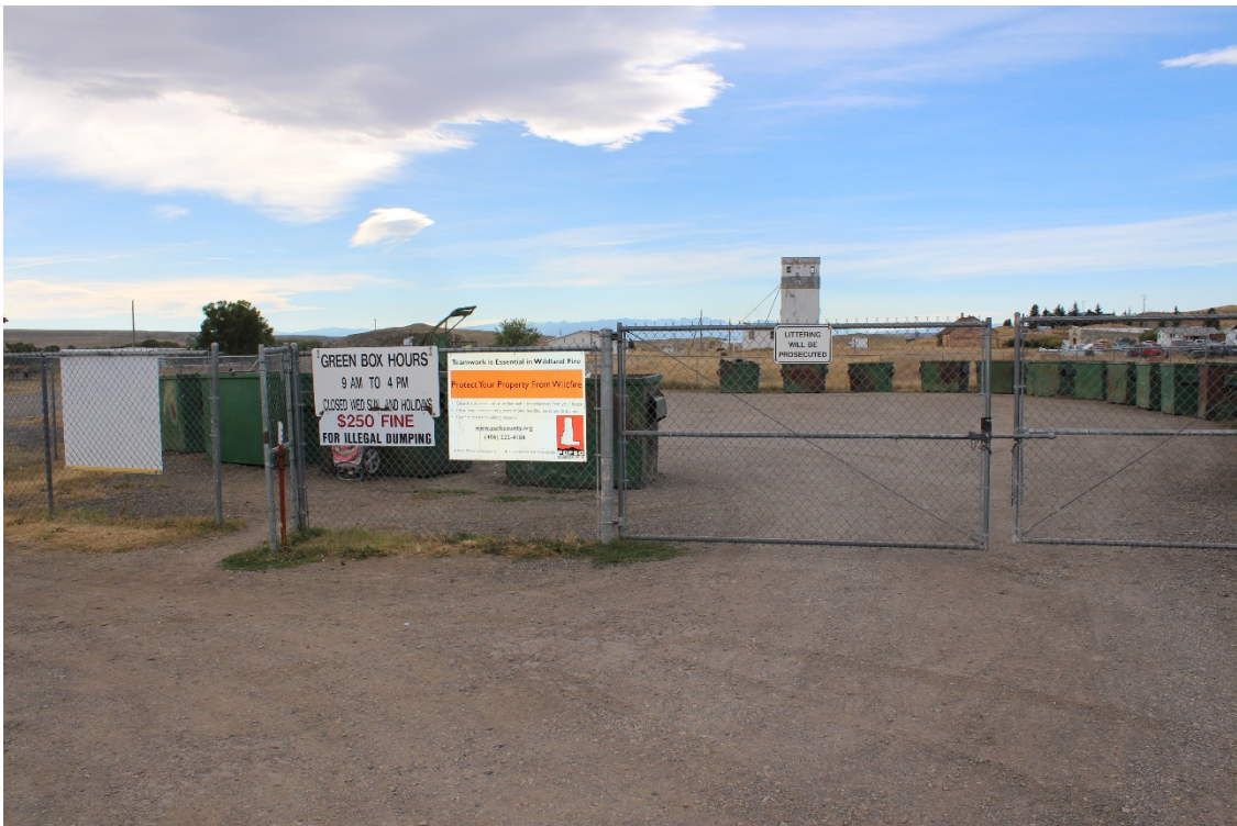
Wilsall Access Gates and Site
