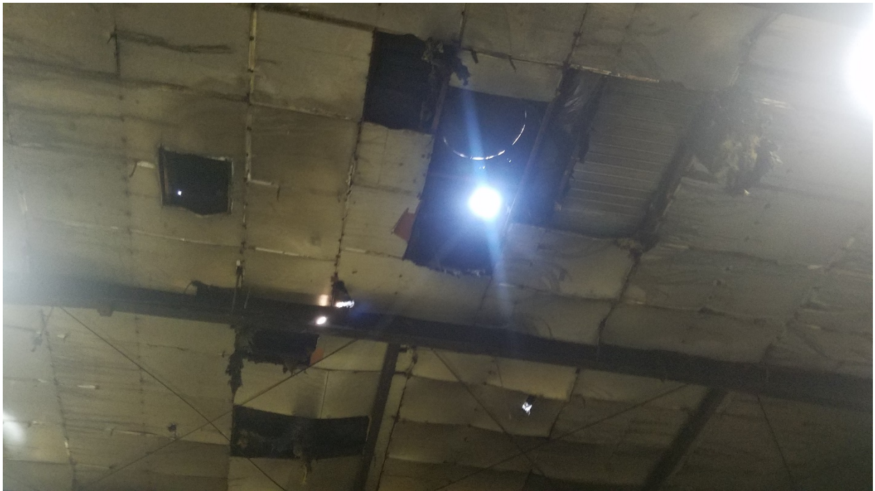
M Street Roof
