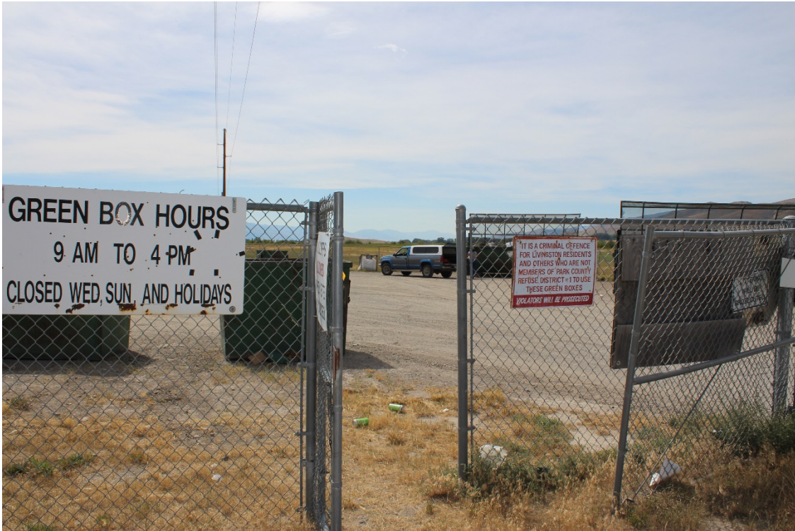
Trail Creek Walk-in Gate
