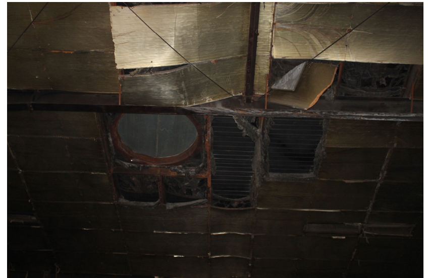
▲ Transfer Station Roof
