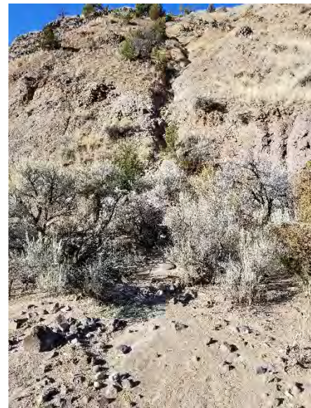
Figure 213 Mile 10.6. Erosion and resulting sediment deposits.
