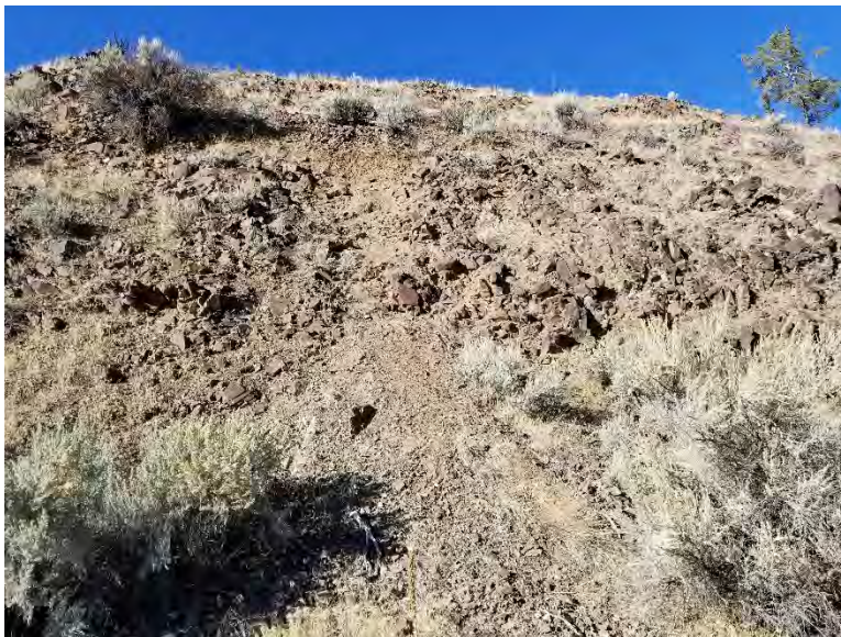
Figure 22 Mile 10.2. Loose Rock.
