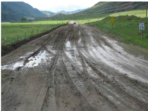
Figure 187 (L) Mile 8.3 looking south on OYTS Road. Drainage is inadequate to handle heavy rains. Photo credit: Alan Shaw; Figure 198 (R) Mile 8.3 Looking south on old railbed.
