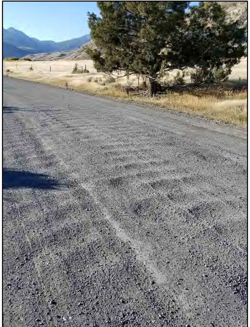
Figure 7 Mile 5.4 looking north.
