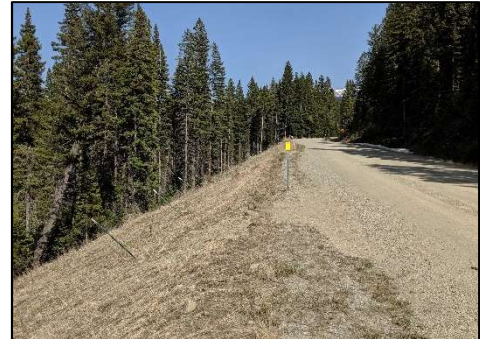
Areas with steep slopes may have an elevated risk of erosion, slope failures, or landslides. Steep slopes also pose a safety risk to drivers as they are difficult to recover from.
