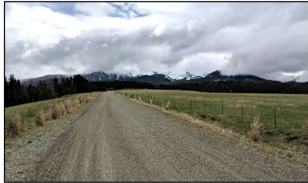
The first 15.7 miles of Shields River Road are paved; the remaining 3.8 miles are gravel surfaced. The majority of the pavement is in deteriorating condition.
